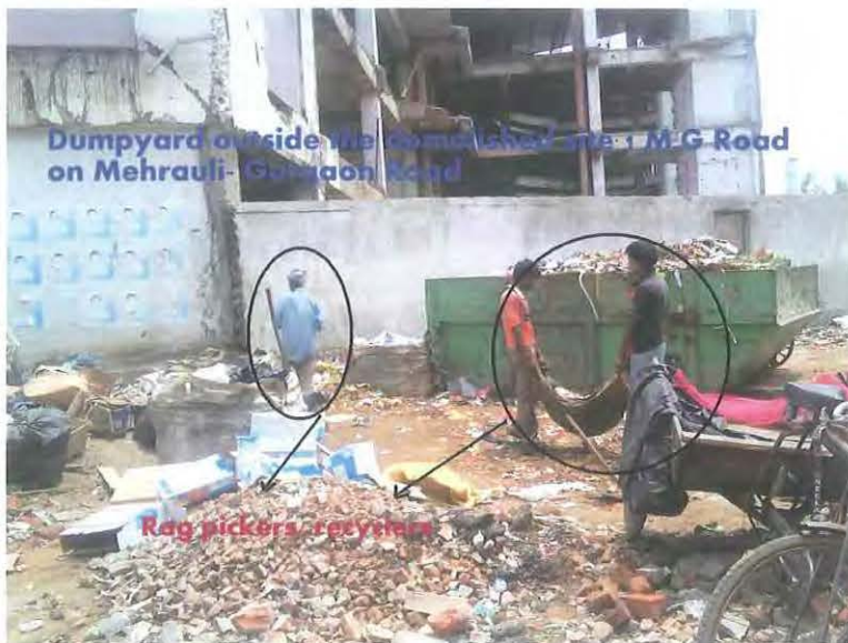
FIGURE 4: STATE OF FILTH AT CHAKKARPUR VILLAGE
