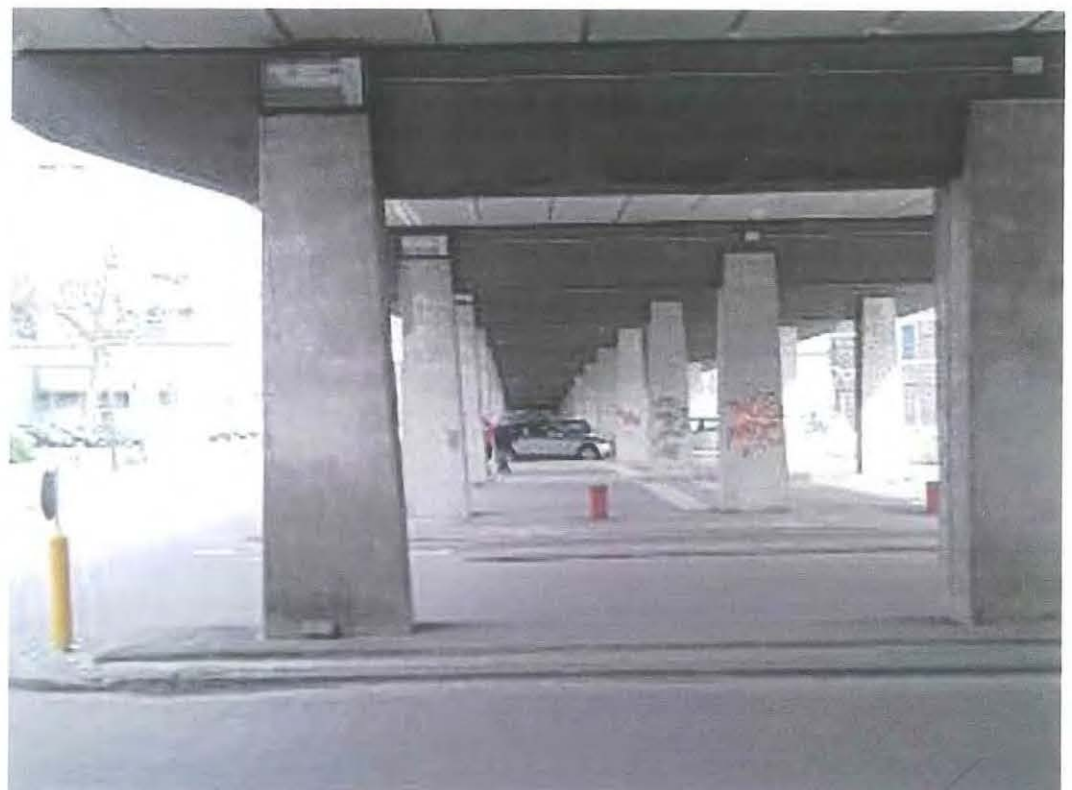
Figure 15: Under the bridge formed by the over passing ring road.
