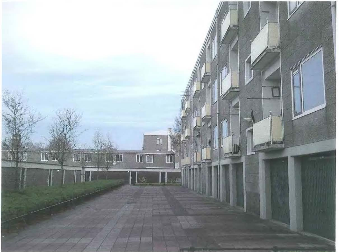
Figure 18: Concealed courtyard behind run- down flats (section 2)
