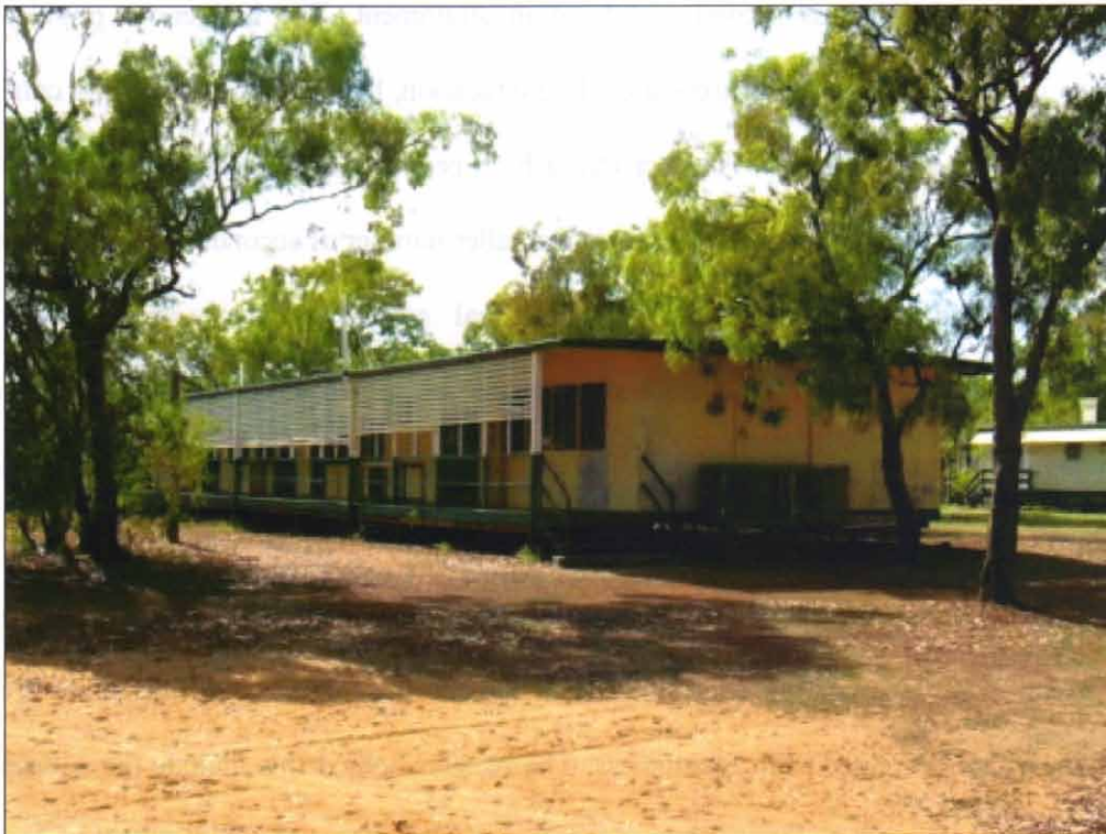
Mornington Island State School, High School block
